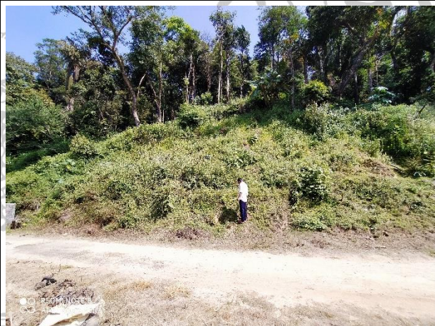
J) Cut slope failure near Biligeri school ( 12^{\circ} 33' 25.50''\text{N}/75^{\circ} 39.96''\text{E} )
