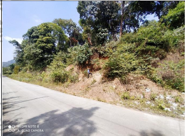
F)Cutslope failure near Shrangalli ( 12^{\circ} 33'6.78''\text{N}/75^{\circ} 47' 3.77'' \text{ E} )
