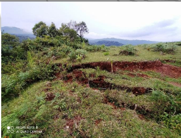
E)Surface cracks and its vertical displacement near kurra motte bane ( 12^{\circ}34' 10.54''\text{N}/75^{\circ}47' 45.25'' \text{ E} )
